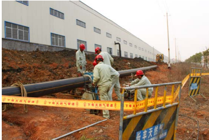
The Construction Site on Xiangdong Ceramic Industry Park
